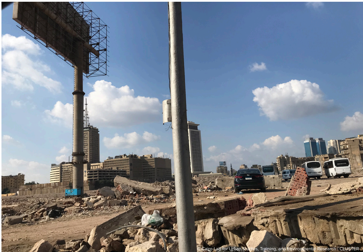
Figure 2 Demolition of informal housing area in Maspero Triangle
