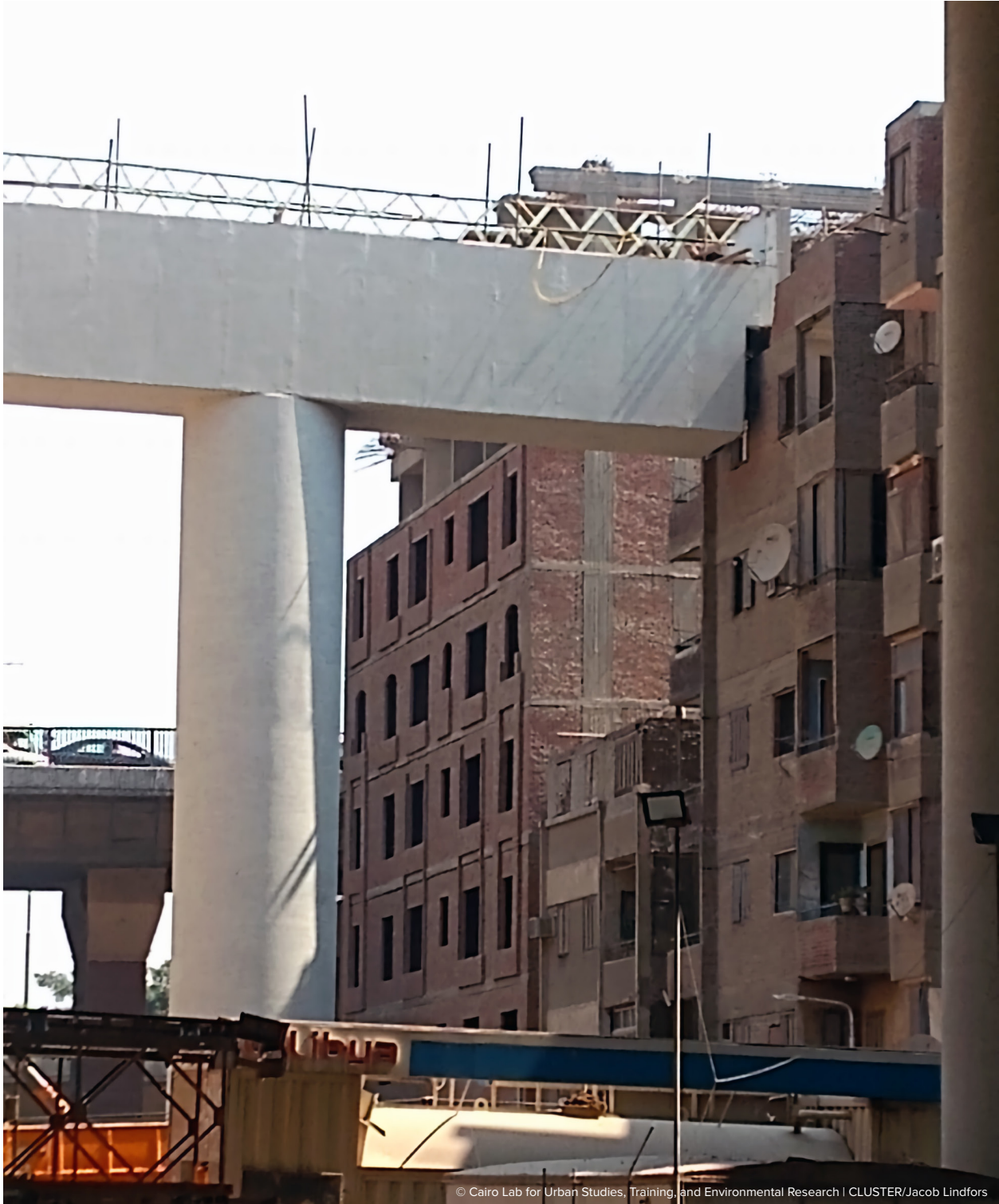
Figure 3 Flyover abutting informal housing
